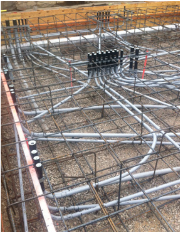
Conduit Installed in a Slab
